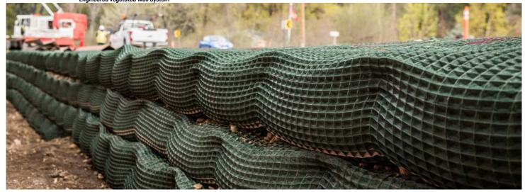
**PYRAWALL™** is an engineered wrap-face vegetated solution for constructing reinforced-soil walls and steepened slopes. The system consists of PYRAMAT® 75 High Performance Turf Reinforcement Mat (HPTRM) and fiber-composite internal bracing. Featuring flexible setback and alignment, PYRAWALL can be customized to unique site conditions and geometrics.
