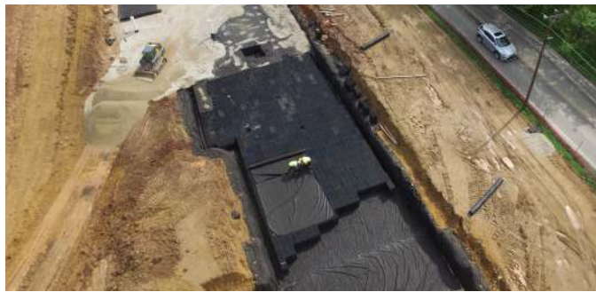
R-TANK SD INSTALLATION
