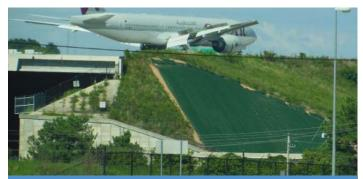
**SOLUTION** ARMORMAX<sup>®</sup> 75 was designed and installed for deep slope stability
