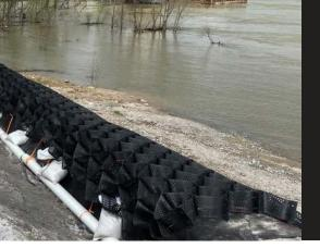
> BaseLok™ GeoCell is a confinement system that can be used on slopes creating a stabilized and permeable layer. We offer an engineered system complete with anchoring components.
