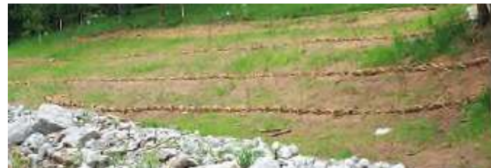
Example of Slope Contouring
