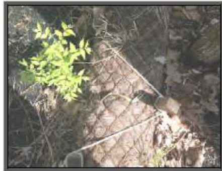
Top View of Laced Coir Logs End to End
