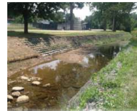
Transition from Coir Log to GeoWeb Wall June 2013
