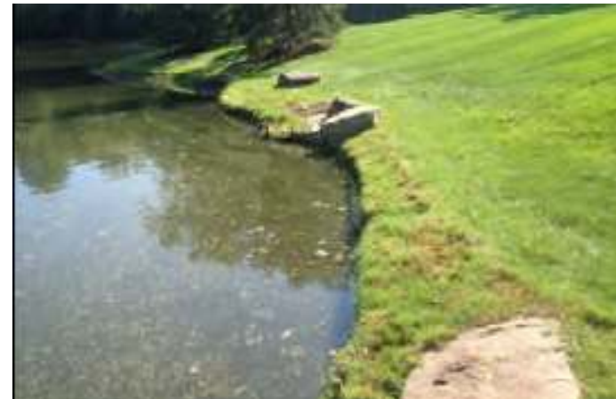
Water's Edge Vegetated with Bent Grass at a Private Residence in Carmel, Indiana (9 years old)
