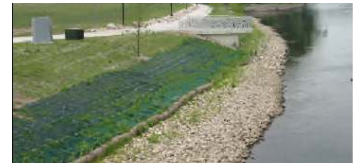
System Solution of TRM, Coir Log & Riprap
