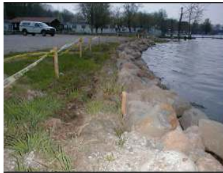
Buried Coir Log at 50%
