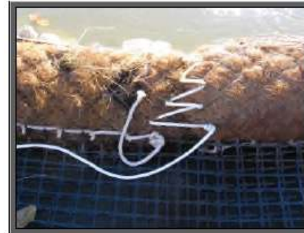
Side View of Laced Coir Logs End to End
