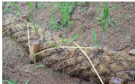
Coir Logs with Standard Staking & Lacing
