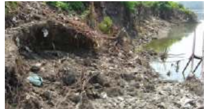
Looking Downstream at Site April 2003
