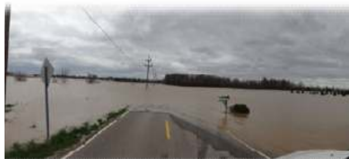
During April 2013 Flooding
