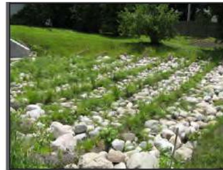
Wedged Coir Log between Logs
