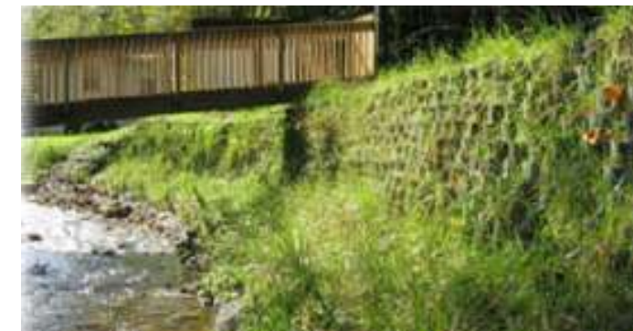
Overgrown 10' GeoWeb Wall with Coir Log at Toe of Slope - Aug. 2012
