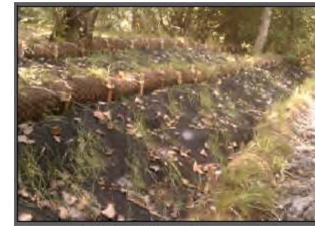
Coir Log Tied to Revetment Structure
