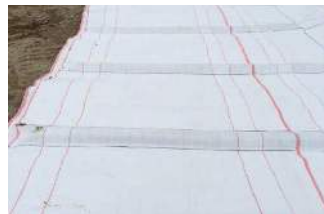
HIGH-STRENGTH FABRIC WITH HIGH TENSILE REINFORCING RIBS
