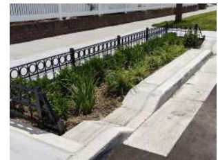
Urban Rain Garden Modular precast T wall system for FocalPoints in tight spaces
