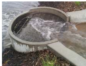
Rain Guardian for curblin pretreatment and energy dissipation
