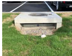
PRETX for larger watershed curblin pretreatment and energy dissipation
