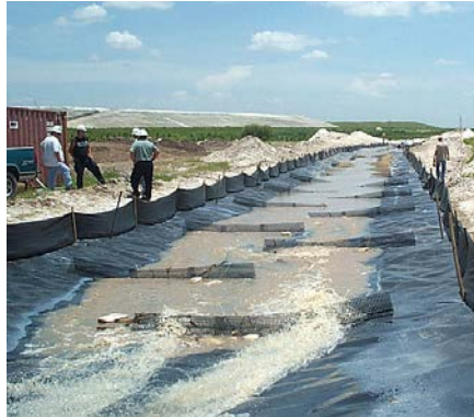
Floc Logs® installed between wattles for increased mixing and reaction.
