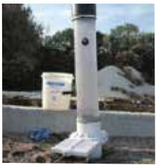
Figure 7: Infiltrator Placement
