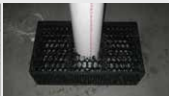
Figure 13: Place inspection port into underdrain module
