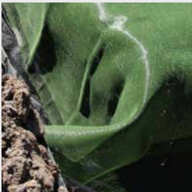
Figure 17: fold corners flat against the tank
