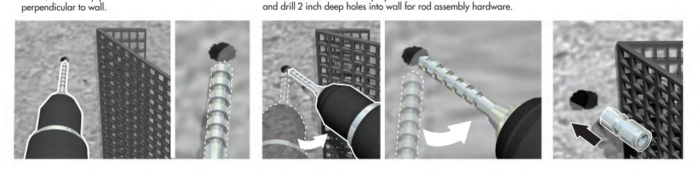
Rotate drill as shown to run perpindidular to Trash Guard Plus
