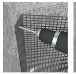
Drill 1/2 inch deep pilot holes into wall at marked areas
