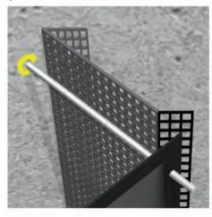
Insert metal anchors into wall.
