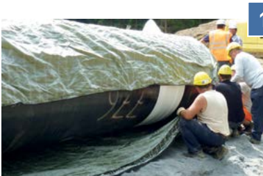
Fixing to pipe section
