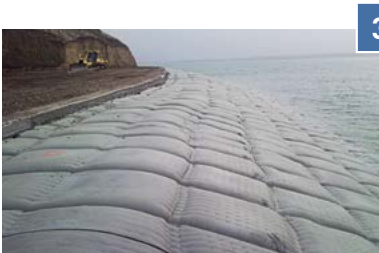
Filling of panels with fluid concrete/mortar
