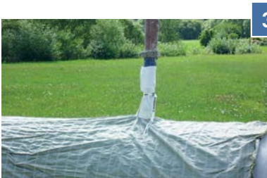
Concreting via filler neck
