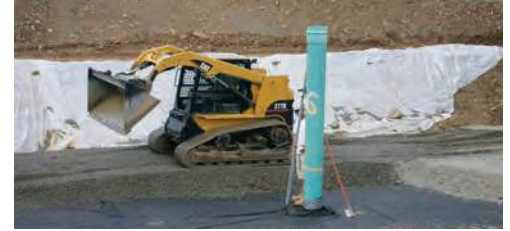
Fig. 18 Use an LGP equipment to place backfill over R-Tank® units.
