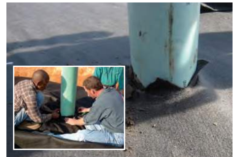
Fig. 14 Cut an "X" into textile to accommodate pipe penetration and seal with a boot
