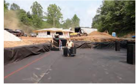
Fig. 5 Use a string line and marking paint to square the system footprint
