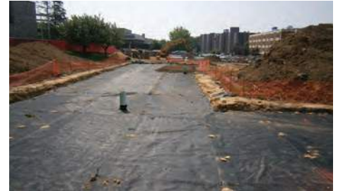
Fig. 19 Overlap geogrid 18" or as required by plans.
