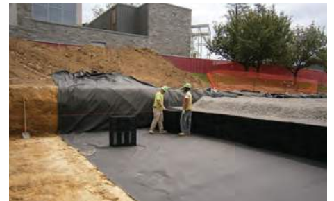
Fig. 3 Pull wrinkles out of geotextiles so material lays flat
