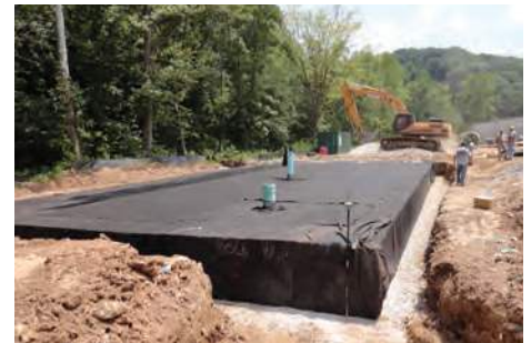
Fig. 15 Finished envelope should lay flat against R-Tank®
