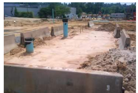
Fig. 22 Secured R-Tank® installation using Jersey barriers
