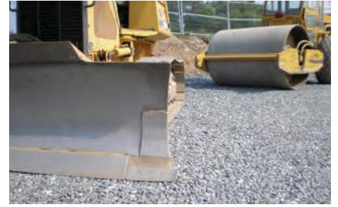
Fig. 2 Base must be smooth to ensure units fit together without gaps
