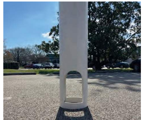
Fig. 10 Inspection port "doghouse" opening
