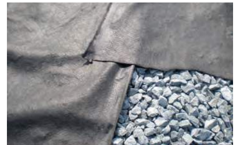
Fig. 4 Reduced overlaps don't create significant savings and can create delays
