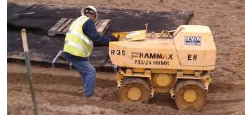
Fig. 17 Vibratory compaction of side backfill is ALWAYS REQUIRED, regardless of what backfill material is used.
