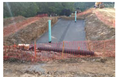
Fig. 21 Secure the installation with temporary fencing
