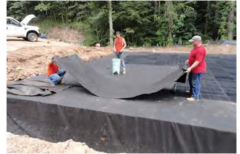
Fig. 13 Encapsulate R-Tanks® with geotextile
