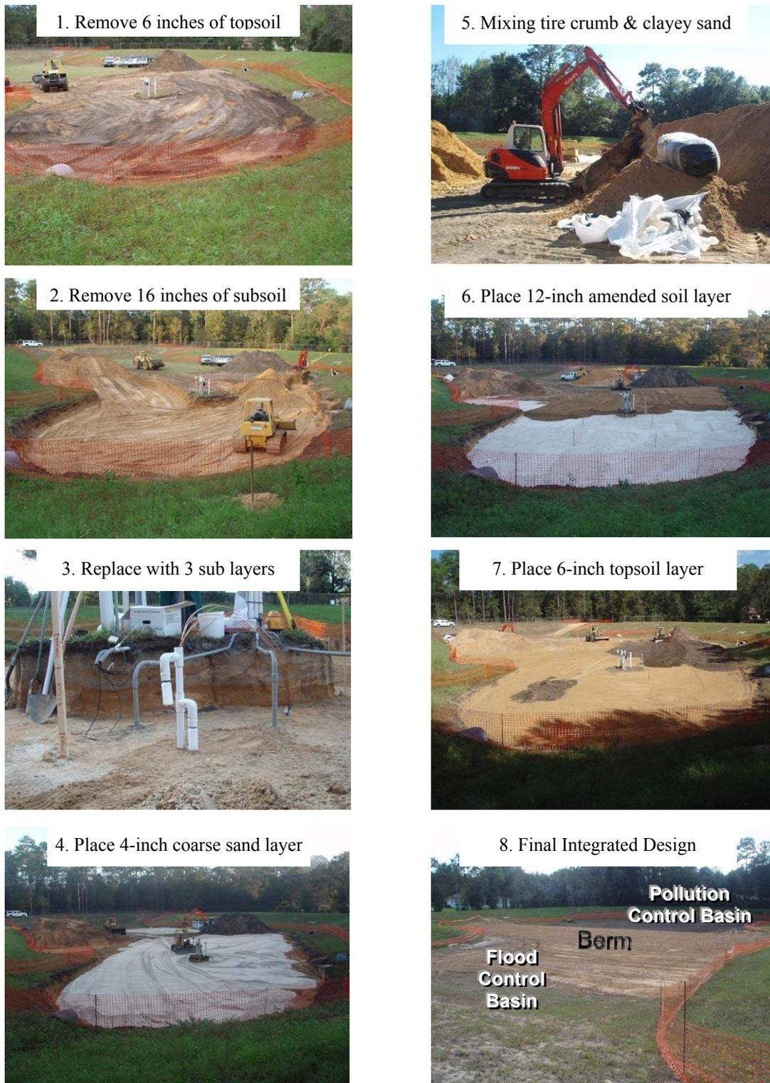
Figure 23 Construction of the new integrated design at the Hunters Trace basin.
