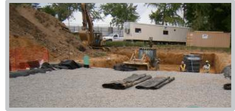
Fig. 18 Use an LGP dozer to push backfill over R-Tank® units.
