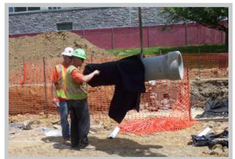
Fig. 16 Install boots onto pipes prior to connecting them to the R-Tank, leaving the clamps loose for final adjustment later
