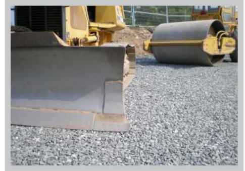
Fig. 2 Base must be smooth to ensure units fit together without gaps
