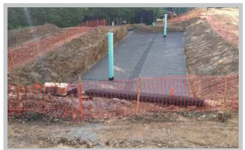
Fig. 21 Secure the installation with temporary fencing
