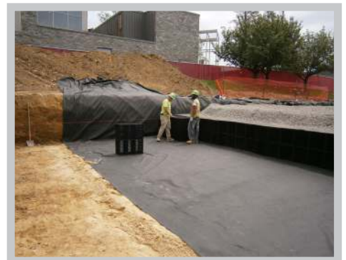
Fig. 3 Pull wrinkles out of geotextiles so material lays flat
