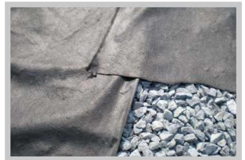
Fig.4 Reduced overlaps don't create significant savings and can create delays
