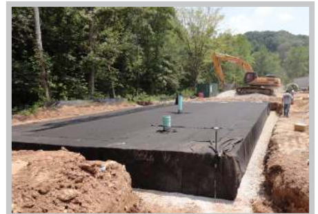
Fig. 15 Finished envelope should lay flat against R-Tank®
