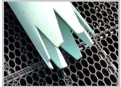
Fig. 9 Cut 8" notches into the bottom of maintenance port
