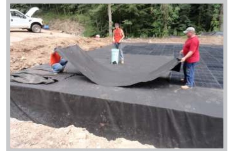
Fig. 13 Encapsulate R-Tanks® with geotextile
