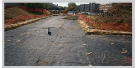
Fig. 19 Overlap geogrid 18" or as required by plans.
