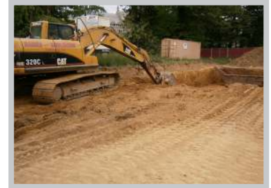
Fig. 1 Excavate according to plans, following all governmental regulations.
