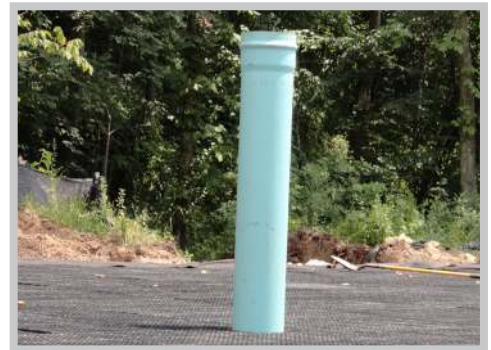
Fig. 10 Installed maintenance port
