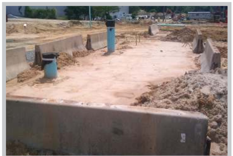
Fig. 22 Secured R-Tank® installation using Jersey barriers
