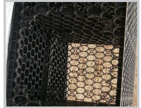
Fig. 11 For HD and SD modules, make space for the pipe by removing the center plate
