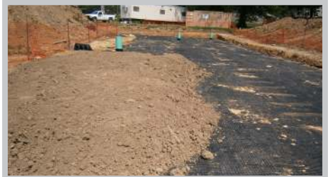
Fig. 20 Pushing backfill parallel to the Geogrid prevents the grid from shoving.
