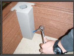
RAIN GUARDIAN PLACEMENT IS SET 26" FROM THE BACK OF THE EXISTING CURB. ENSURE THE CONCRETE BASE EXTENDS AT LEAST 4" BEYOND THE FILTER WALL TO SERVE AS A SPLASH DISSIPATER. APPLY ADHESIVE TO BASE OF RAIN GUARDIAN AND POSITION ON CONCRETE BASE. USE ADDITIONAL ADHESIVE AROUND BASE OF INTERIOR TO ESTABLISH WATER-TIGHT SEAL. USING PILOT HOLES IN CORNER POSTS, DRILL 3/16" HOLES INTO CONCRETE WITH 6 1/2" MASONRY BIT AND HAMMER DRILL. SECURE WITH 1/4" x 5" MASONRY SCREWS (PROVIDED).
