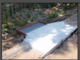
FILL VOID BETWEEN EXISTING CURB AND RAIN GUARDIAN. INSTALL FRAMING TO PREPARE FOR CURB-CUT AND APRON INSTALLATION. SIDES OF APRON SHOULD BE RAISED SIGNIFICANTLY TO BLEND INTO CURB AND MATCH TOP HEIGHT OF RAIN GUARDIAN SIDE DEBRIS WALL.
