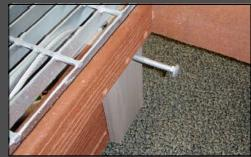
When pouring the concrete inlet, ensure the carriage bolts on the Rain Guardian are surrounded by at least 2" of concrete on all sides. The top of the Rain Guardian grate will be 10.5" above the top of the concrete base and 1.5" below the rain garden overflow elevation to accommodate a sloped apron from the gutter to the Rain Guardian.
