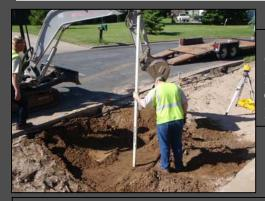
EXCAVATE 16" BELOW THE DOWNSTREAM GUTTER ELEVATION (I.E. THE RAIN GARDEN OVERFLOW ELEVATION) TO ACCOMMODATE THE 4" CONCRETE BASE. THEREFORE, THE TOP OF THE CONCRETE BASE IS 12" BELOW THE RAIN GARDEN OVERFLOW ELEVATION.
