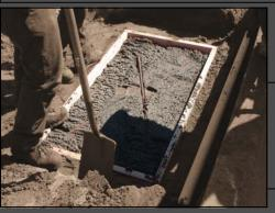
REBAR IS PLACED DIAGONALLY AFTER 2" OF CONCRETE HAVE BEEN POURED TO PROVIDE REINFORCEMENT OF THE CONCRETE BASE.
