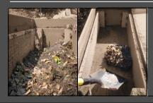
SEDIMENT, LEAVES, AND GRASS CLIPPINGS TRAPPED INSIDE THE CHAMBER ARE EASILY REMOVED BY THE LANDOWNER WITH A SHOVEL. THE DROP-IN FILTER WALL CAN BE EITHER SWEPT CLEAN OR RINSED WITH A GARDEN HOSE TO MAINTAIN OPTIMAL FILTRATION CAPACITY.
