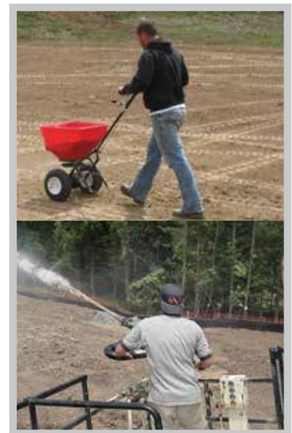
APS Siltstop powder can be applied dry by a number of different methods, either by itself or cut with dry sand, depending on equipment and project considerations. APS Siltstop powder and emulsion can be hydraulically applied along with seed, mulch and fertilizer.
