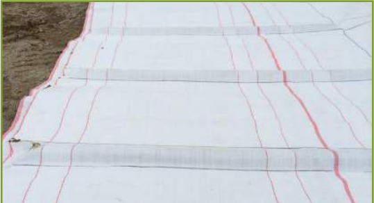
High-strength fabric with high tensile reinforcing ribs
