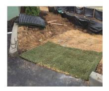
**ShearForce12** eliminates soil erosion at flow-induced shear stresses above 12 lbs/sf and **provides permanent erosion protection** that meets or exceeds that of 36" rock rip rap.
