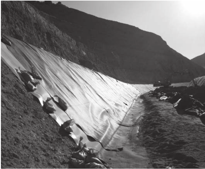
Fabric shall have the proper overlap and be free of any holes or tears.
