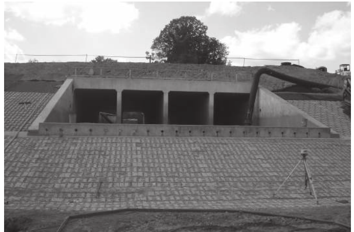
Backfilling should occur as early as possible to protect the filter fabric from UV damage.
