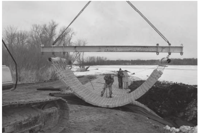
To assist in aligning the unit being placed, use of a pry bar may be necessary.
