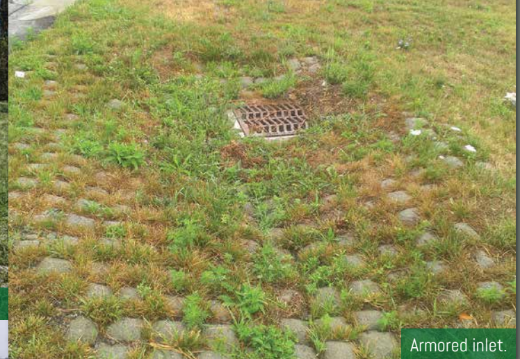
Outlet armored with Flexamat®, 3 years after installation.
