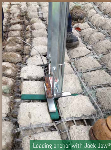
Gas powered driver installation.
