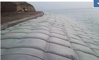
Filling of panels with fluid concrete/mortar
