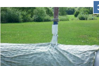
Concreting via filler neck
