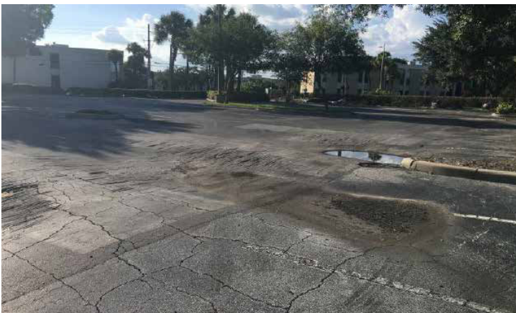
Prior to installation
