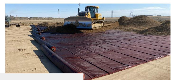
Double layer construction provides varied pore sizes for excellent separation and superior filtration and flow characteristics of a fine to coarse sand layer.
