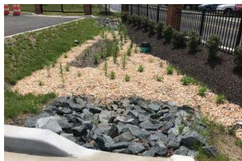
Curb riprap (lot A)
