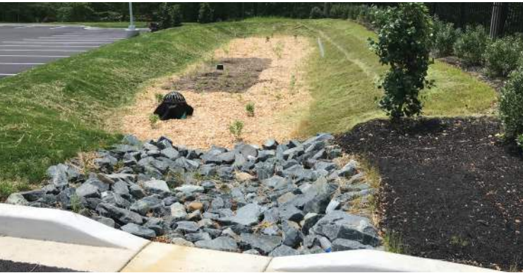
Riprap inlet to FocalPoint planted system (lot N).
