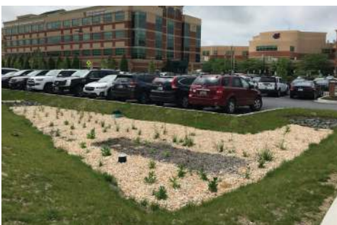
FocalPoint post-installation (lot A)
