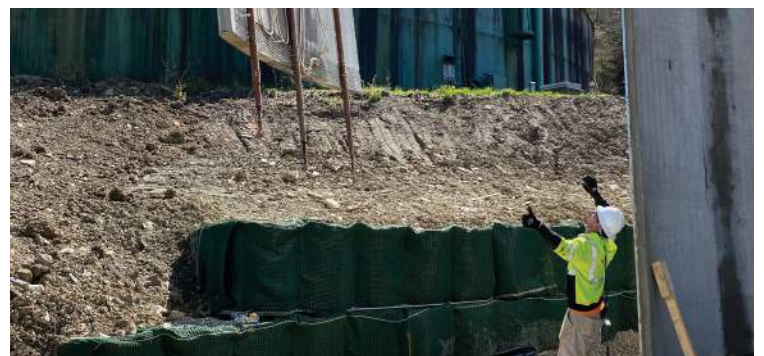
Placing of water tank panels near Scourlok face.
