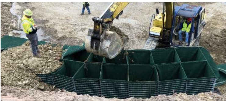
First layer of Scourlok being filled - 2 cells deep.
