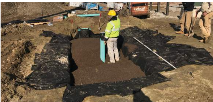
Access created for water tank installation.
