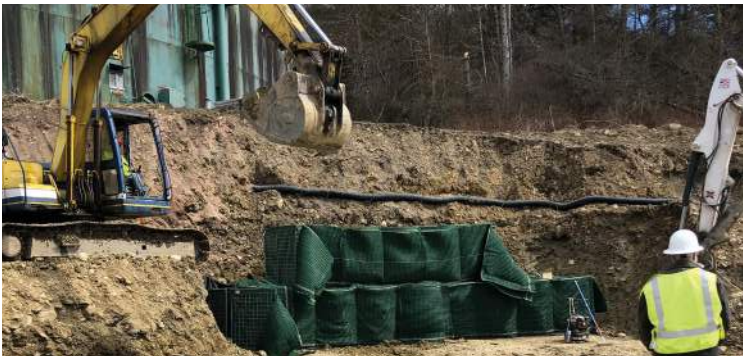
Machinery filling cells with on-site material.
