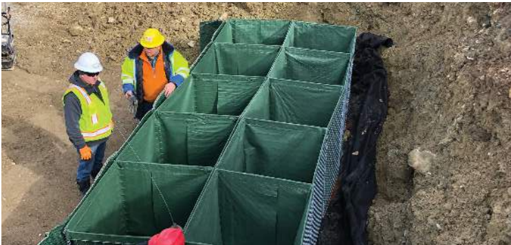
Connecting the cells for the first layer of Scourlok.
