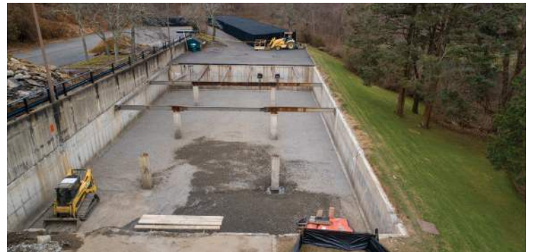
Base prep for the installation of the system.
