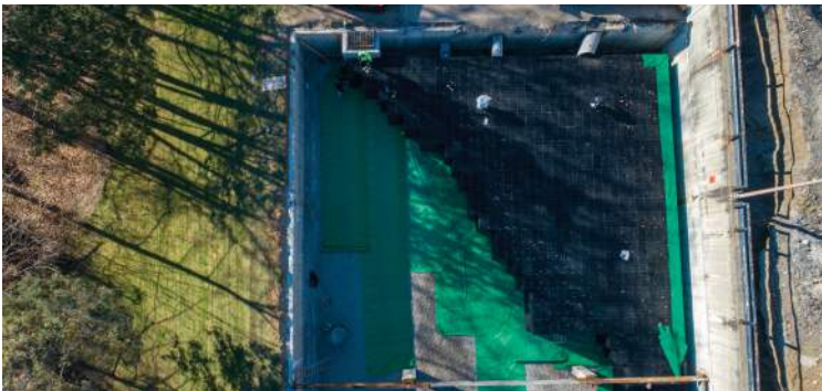
R-Tank HD Pent 7-ft modules filled the existing concrete footprint.
