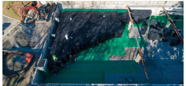
The system was wrapped in SR-18 microgrid (pictured in green).
