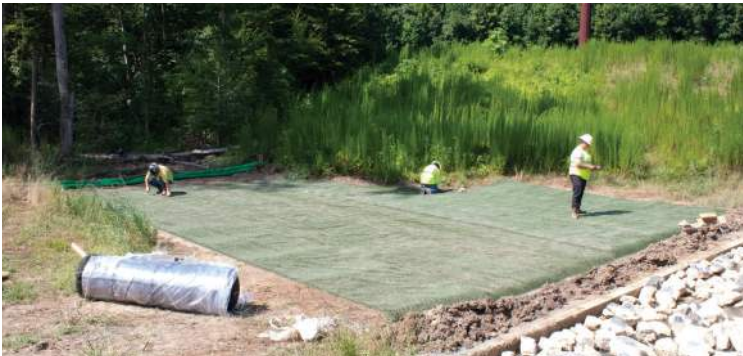
Before hurricane—emergency spillway.
