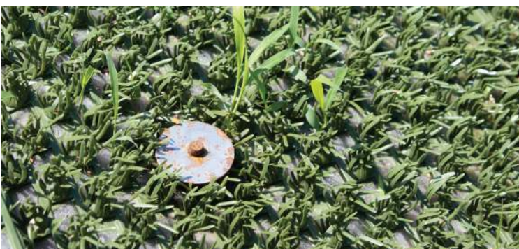
Anchored using pins and washers.
