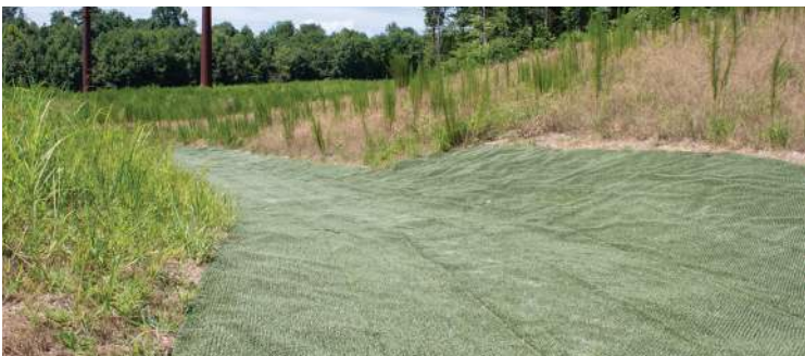
Before hurricane—outfall channel.
