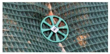
Complete Engineered Earth Anchors installation, with anchor flush against Pyramat.
