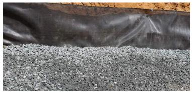
Installation of trench drain using geosynthetic fabric to protect from seepage.
