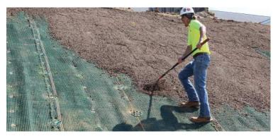
To promote vegetation, seed was placed beneath Armormax, beneath evenly spread soil coating and above soil coating.
