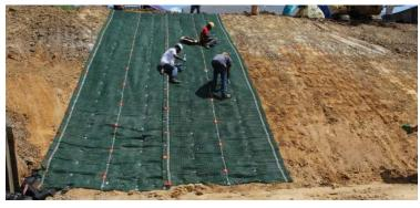
Beginning of Armormax install with Pyramat rolled down the hill and washer pins installed.
