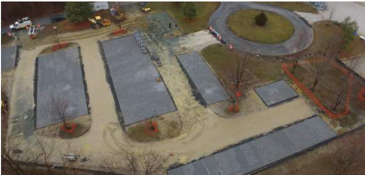
Parking lot under construction.
