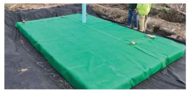
Modular underdrain installed inside geotextile envelope along with the maintenance port.
