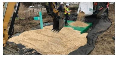
Microgrid mesh installed, then the top and sides backfilled with peagravel.
