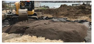
High performance biofiltration soil installed.
